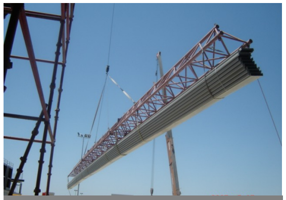
Lifting of panels
