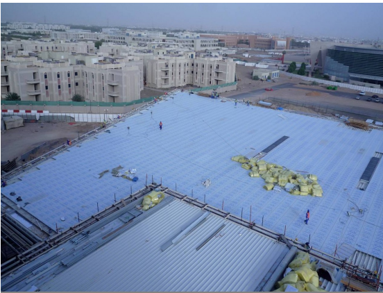
Installation in Progress
