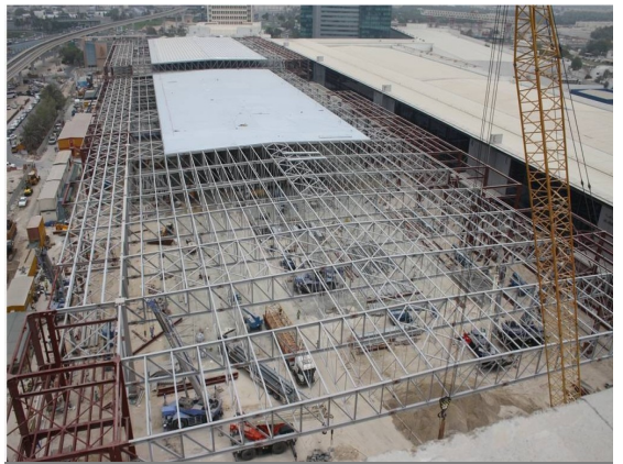
Installation in Progress
