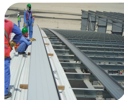
Roll Forming onto the Roof
